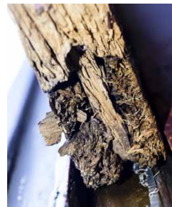
Photo 45: Lower corner joint of lower sash at window #29. The base of the stile has rotted off but the tenon of the rail appears to remain intact. Most lower sash corner joints are in better condition.
