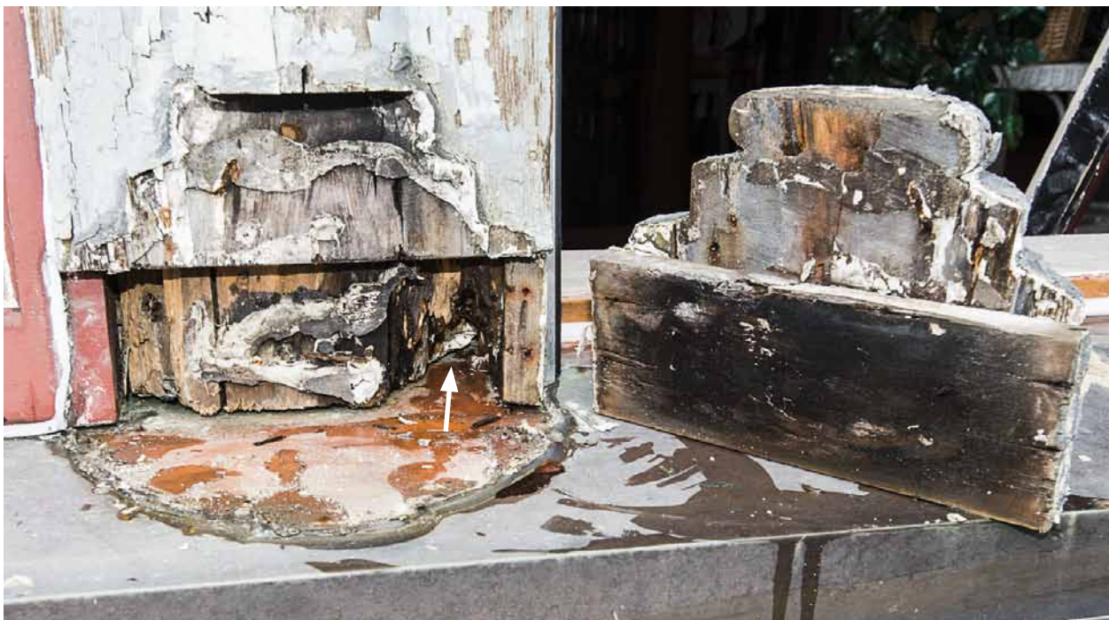
Photo 13: Turned base to the pilaster between windows 22 & 23 removed showing rotted wood on the right side behind it along with water that had leaked in. The arrow points to where the flashing is not turned up allowing water to get into wall under the window and the hall ceiling below.
