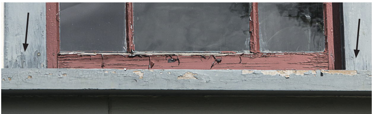
Photo 41: Detail of window #36 showing the weather checking of the bottom rail of the lower sash that warrants conservation with epoxy consolidants. The corner joints were found to remain firm. The arrows point to moderate splits at the base of the side casings that can readily be treated with epoxy consolidants. The sill was found to be in sound condition other than peeling paint.
