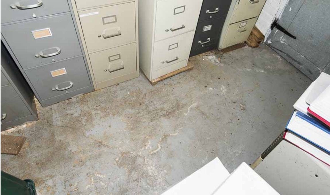
Photo 102: Room below the Town Clerk's office showing stains from past dampness or leaks. No signs of current leaks were observed.
