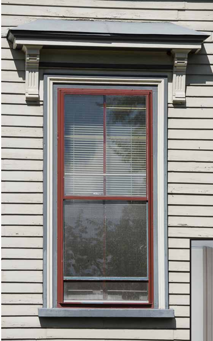
Photo 51: Window #16 (type A) on the south facade. All the first floor windows are of this type, and all are fitted with aluminum storm windows. The storms have protected the sash from the extensive glazing deterioration and weather checking that is present on most of the upper floor sash. The sills are also in sound condition. The projecting window heads are covered with sheet metal. As the storm windows are at least 20 years old, they are not as tight as new storms would be, and they tend to be cranky to operate.
