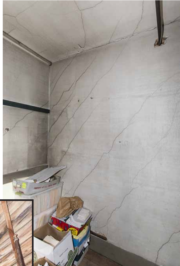
Photo 86: Room in the southeast corner of the balcony level that is now used for storage. Its plaster walls have not been painted or otherwise repaired for many years and therefore show the cracks from the long past structural movements of the tower.
