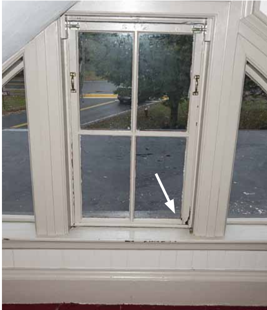
Photo 14: Interior side of window 23, which is removable from the interior to access the entry porch roof. The arrow points to its severely rotted lower corner.
