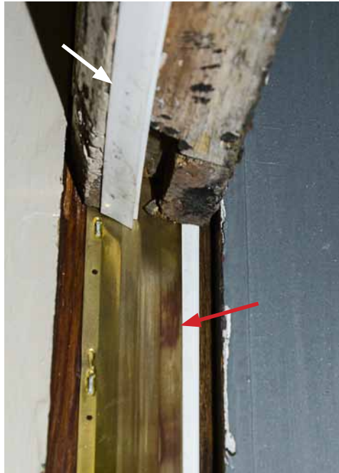
Photo 53: Typical weather stripping on the first floor lower sash. The white arrow points to the vinyl leaf used on the underside of the lower rails of the lower sash. The red arrow points to the single leaf spring bronze used in the jambs. Both types are not very effective.
