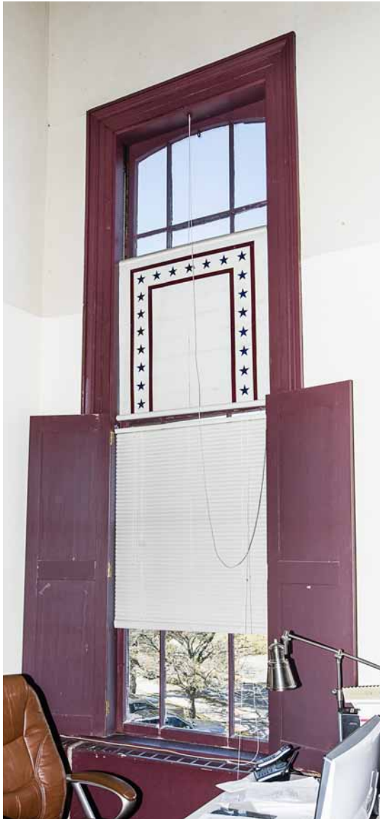
Photo 42: Interior of typical type B windows located in the former meeting hall space. The shutters are modern additions.
