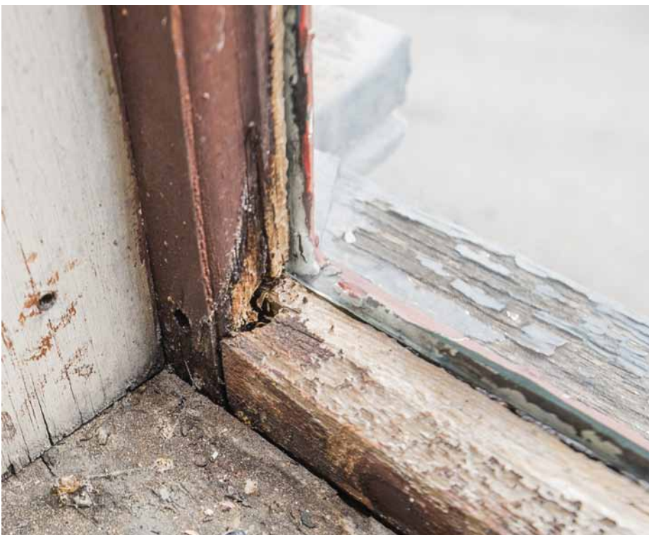
Photo 50: Window #40 (type D). The top interior surface of its bottom rail is severely eroded from years of condensation draining off the glass, and there is substantial separation at the corner joint. At minimum the corner joints need to be tightened; replacement of the bottom rail may be warranted due to the erosion.
