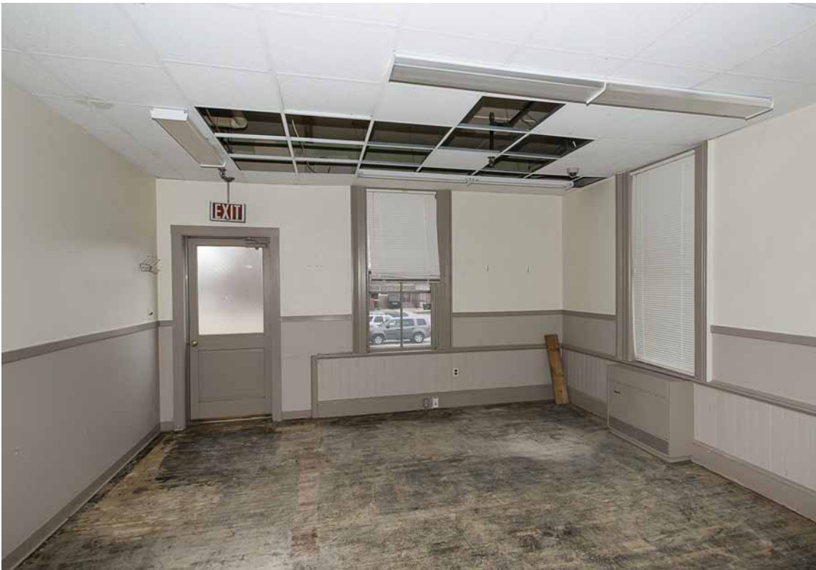
Photo 70: The treasurer's office at the southwest corner of the first floor after it was cleared out due to being flooded from a frozen pipe. The vinyl-asbestos tile has been removed showing the original wood floor, and wood wainscot.
