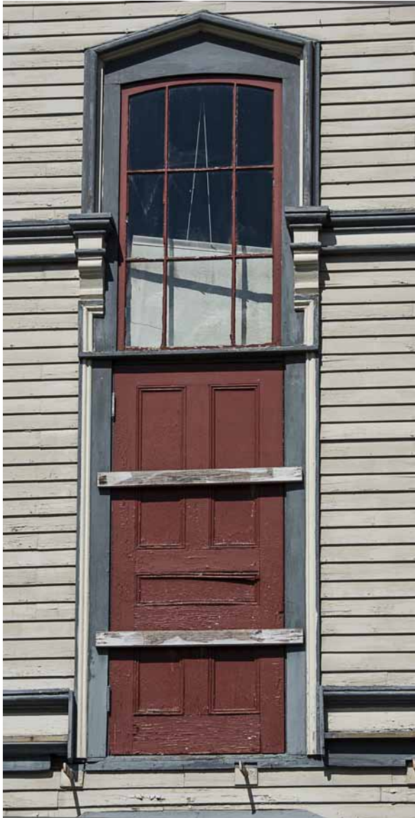
Photo 26: South facade window #34 with obsolete egress door having replaced the lower sash. In 2003 this window area was left as is without the repairs done to the other facade pending the development of plans for an addition to this side. Planning for a possible addition has recently been revived.
