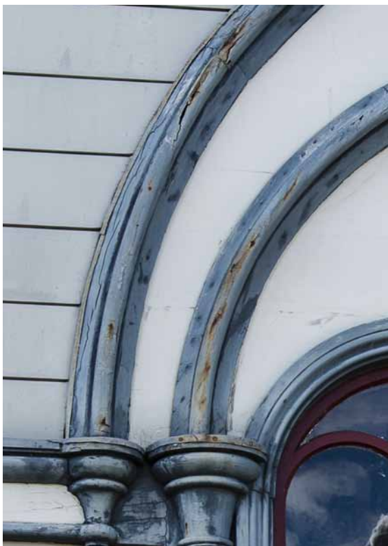
Photo 18: Arched trim above window 42 has substantial cracks, probably started by rusting nails. The outer trim is substantially worse than the inner one. The turnings below the trim appear to be sound and are capped with copper.
