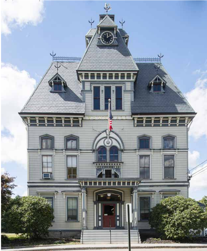
Photo 3: Front (east) facade. All the rusticated boarding on this facade was replaced in 2003 with western red cedar over battens to create an air space behind the siding. The siding remains in good condition other than worn paint.
