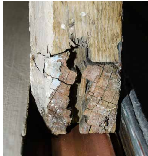
Photo 54: Common defect at the corner joint of a lower sash looking up at the bottom of the stile and rail. The joint remains solid, but the portion of the stile that covers the rail tenon has fallen away and the end grain at the bottom of the stile is checked. This condition is easily repaired with epoxy conservation.
