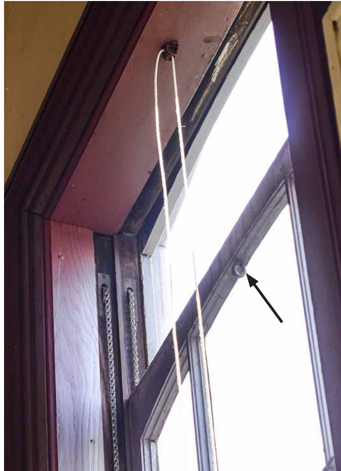
Photo 43: Detail of typical type B showing the weight chains and pulleys in good condition for both the upper and lower sash. The arrow points to a metal loop formerly used to operate the upper sash with a long pole. Currently the upper sash are not opened.
