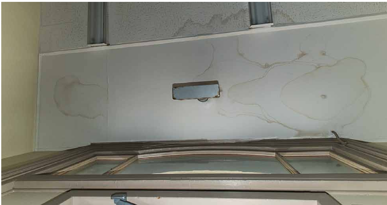
Photo 11: Ceiling in front entry hall above the front door has water damage from chronic leaks that appear to stem from the defective flashings and woodwork at the window directly above that is shown in photo #10. The leaks occur only during prolonged periods of wind driven rain.
