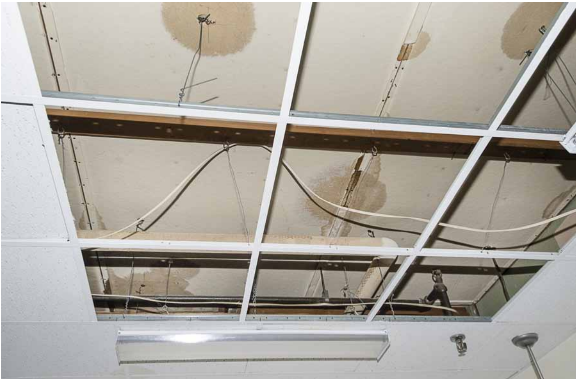
Photo 66: Detail showing that the ceiling above the acoustic panels is fiberboard that covers whatever remains of the original plaster ceiling.
