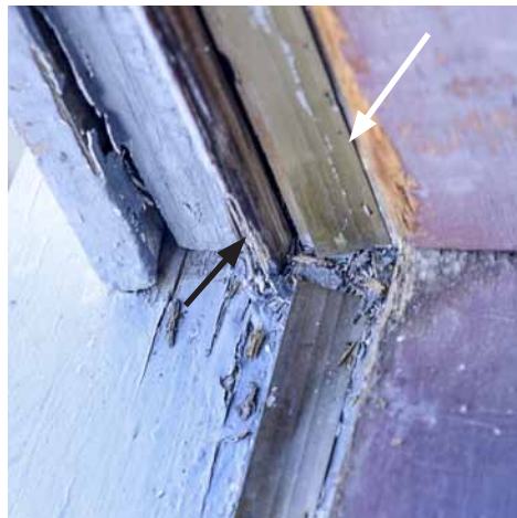
Photo 42: Interior of typical type B windows located in the former meeting hall space. The shutters are modern additions.
