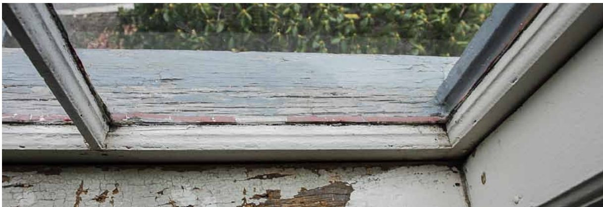
Photo 48: Windows#20 (type C). Other than the glazing the sash is sound. Its sill has moderate weather checking, but its wood remains sound and firm. The checks can be filled with an epoxy filler. Most sills were found to have little or no checking.
