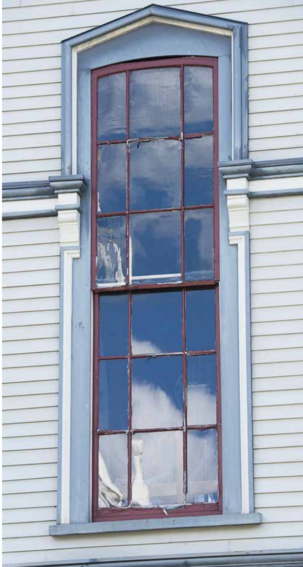
Photo 37: Window #32 on the north facade. This window is one of the most deteriorated ones in the building. The meeting rail of the upper sash has dropped down almost an inch and an inch has been added to the bottom of the lower rail of the lower sash. The window is in the stage area of the original meeting hall. It was originally varnished, but has not been refinished since about 1900. As a consequence, its interior surfaces are deeply eroded from years of water damage from condensation running down off the glass. There is extensive failure of the glazing compound, which is typical of most of the 2nd floor windows, and it also retains most of its original glass. In other respects its condition is far worse than most of the 2nd floor sash.
