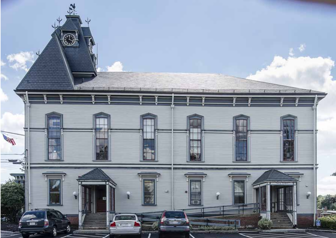
Photo 5: North facade. All the clapboards were replaced in 2003. There are numerous defective mortar joints in the access ramp that need to be cut out and repointed as well as some in the foundation.
