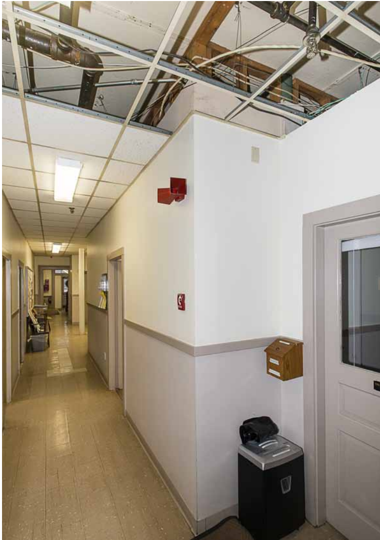
Photo 63: The main first floor corridor at its west end looking east towards the front entry. The dropped ceiling panels have been removed to repair a frozen pipe that flooded the treasure's office. The wall framing above the dropped ceiling shows that the corridor walls are of relatively modern construction. The pipes for the sprinkler system are visible above the ceiling panels.
