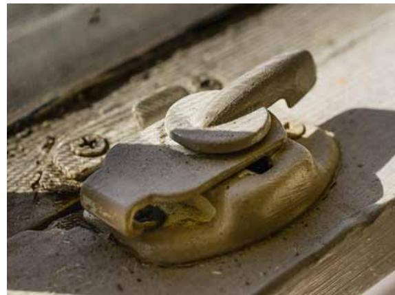
Photo 56: Typical original sash lock. A relatively small number of windows retain their original locks in functional condition.
