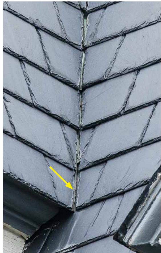
Photo 29: Copper flashings at the closed valley marked with the yellow arrow in photo 28 appear to be worn with areas of holes (arrow). Leaks appear on the roof sheathing in the attic only during periods of prolonged heavy rain with strong NE winds. See photo 87.
