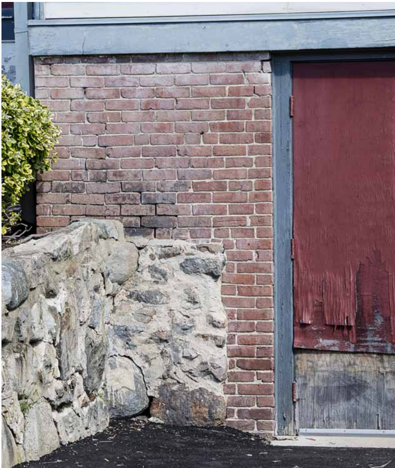
Photo 23: Typical area of defective mortar joints on the rear facade foundation. The deteriorated plywood door has been replaced with a modern metal door since this photo was taken.
