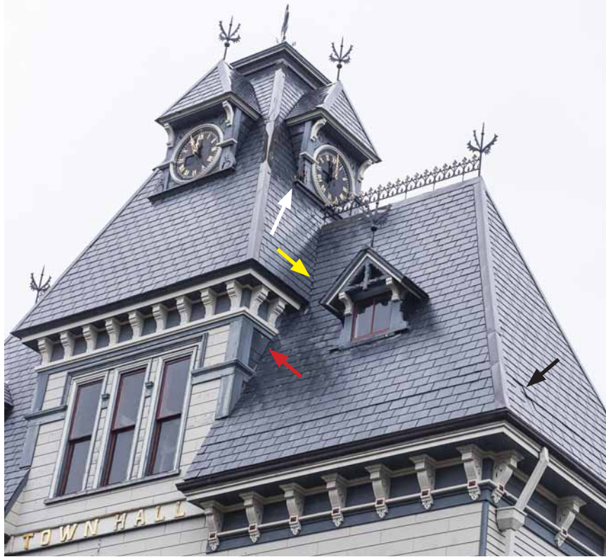
Photo 28: Overview of the front facade tower roofs. The slate is black Monson that is largely in good condition. The gutters were replaced in 2002. The arrows point to defects shown in the following photographs. The horizontal shadow line at the base of the slates four courses up from the gutter reflects the limit of slates removed and reinstalled to replace the gutter in 2003. It is not a defect.
