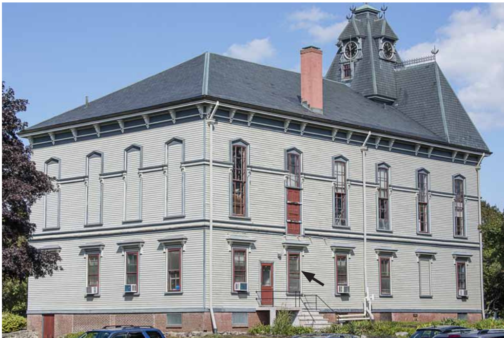
Photo 2: Rear (east) and south side facades. The chimney was recently rebuilt with cement block. The arrow points to a window that replaced an original door that is visible in historic photo 1.
