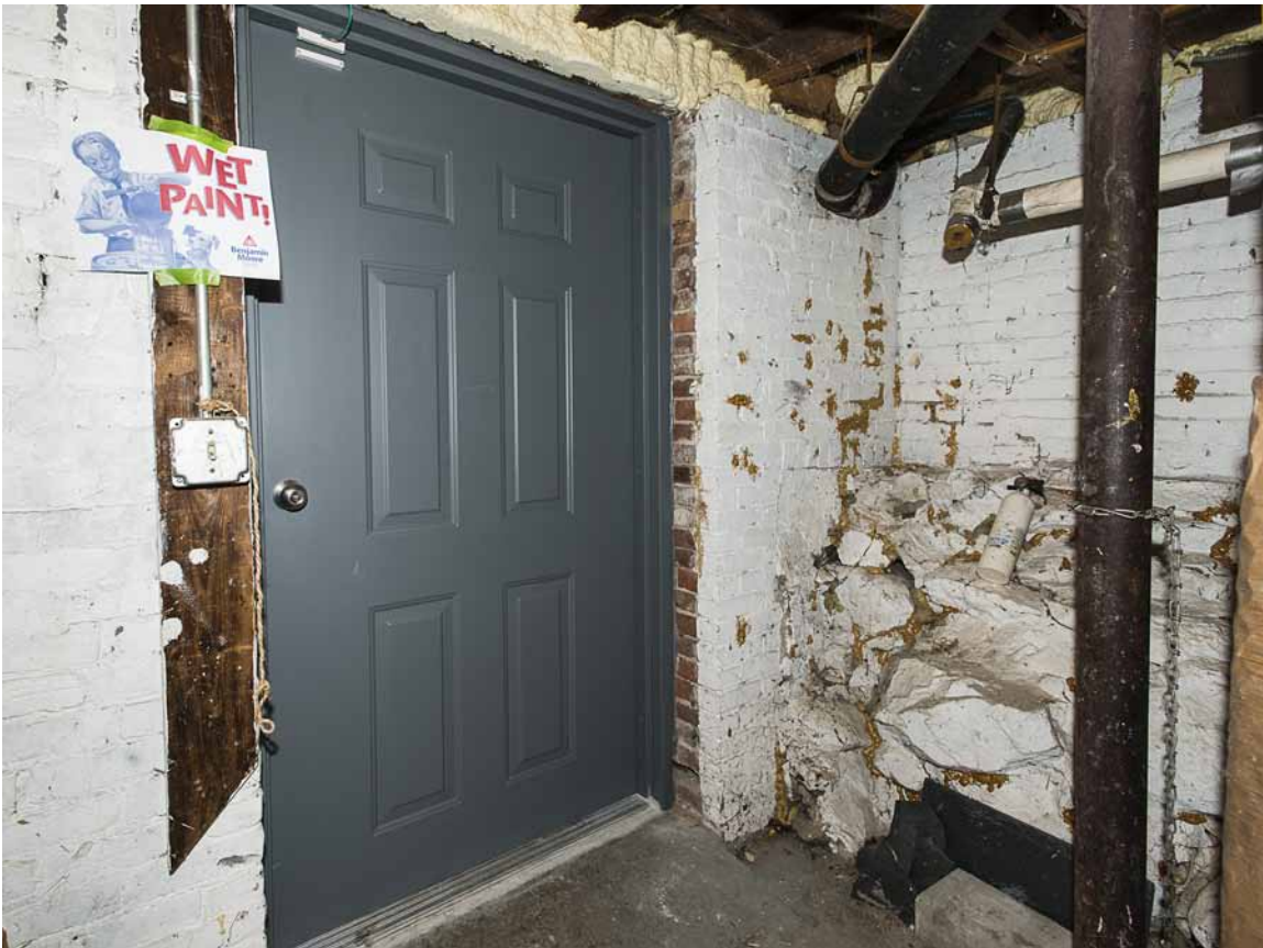
Photo 103: Northwest corner of basement with modern metal door leading to the outside. Foam has been used in an effort to seal the walls from water and outside air intrusion.
