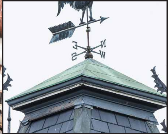
Photo 93: Top of clock tower and base of weathervane. The penetration of the weathervane shaft is a likely source of the leaks in photo 94, but there may be other defects in the copper roof and cornice woodwork.
