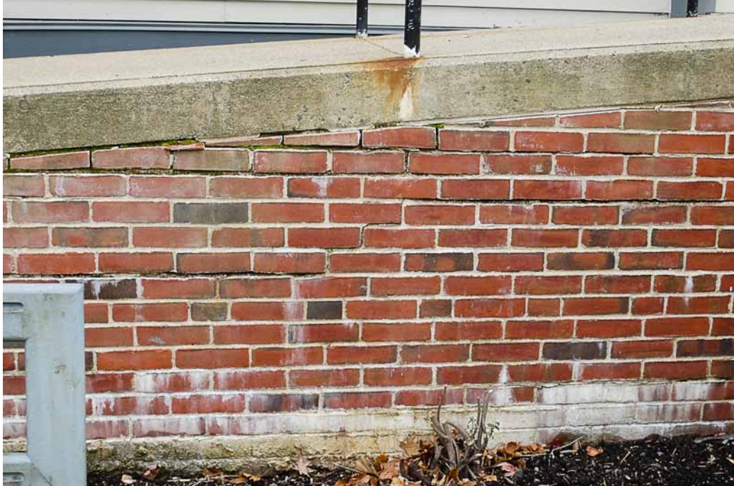
Photo 22: Defective mortar joints at the access ramp.
