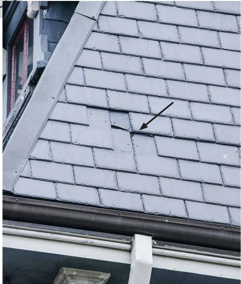
Photo 32: Broken slates exposing felt paper at the location marked with the black arrow in photo 28. Despite the breaks there do not appear to be any leaks associated with this condition.
