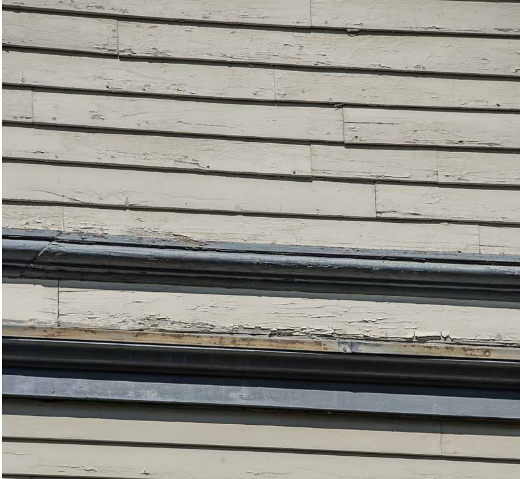
Photo 24: Clapboards on south side facade were not replaced in 2003. They have extensive paint failure and some splits at the butt joints. They appear to be original. The lower belt course is clad with sheet metal that still appears to be serviceable. The upper one is not clad (see photo 25).
