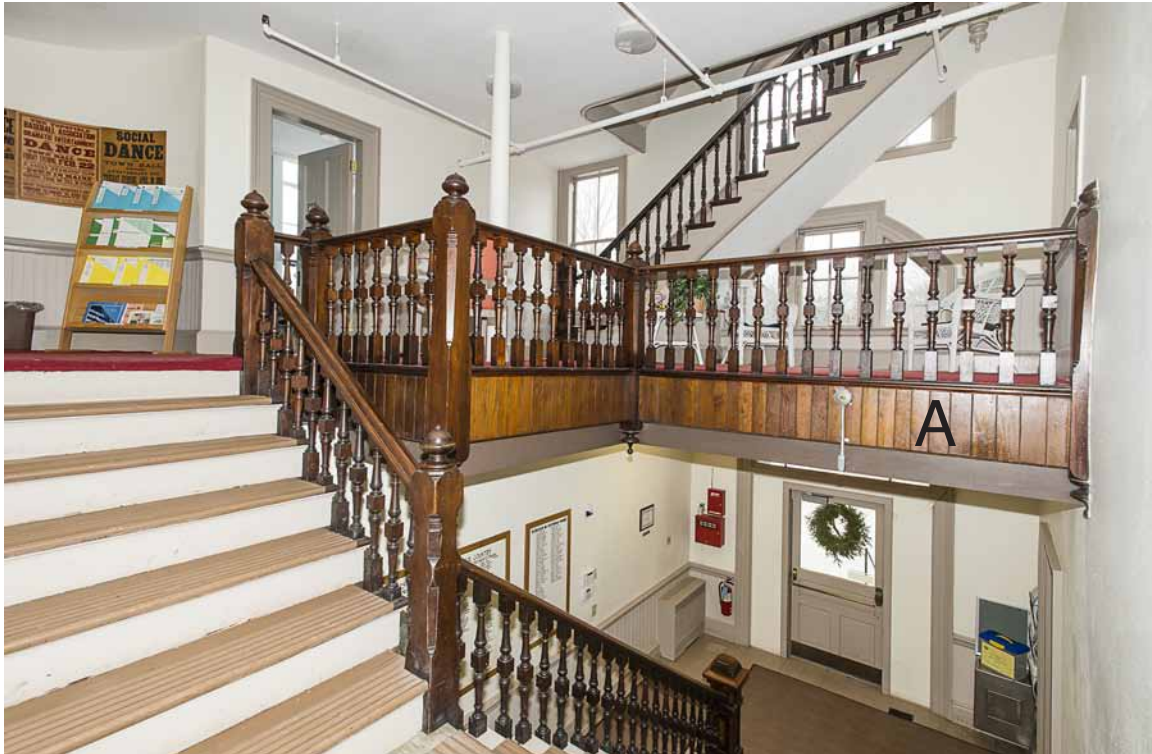
Photo 73: Second floor landing of the front stair looking towards the front of the building. This space retains its original woodwork. The height of the wood facing marked “A” may reflect the original thickness of the floor structure with the tan band below reflecting a past lowering of the ceiling.
