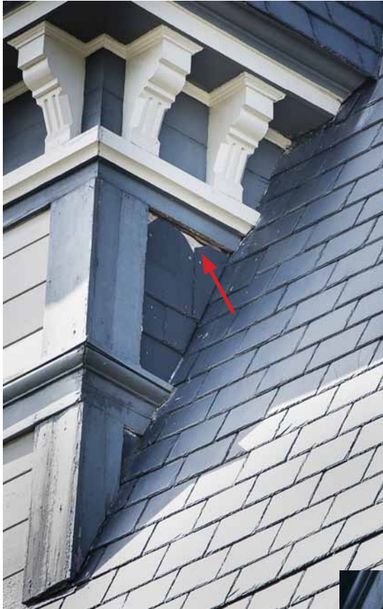
Photo 31: Broken slates exposing wood sheathing at the location marked with the red arrow in photo 28. Despite the breaks there do not appear to be any leaks associated with this condition.
