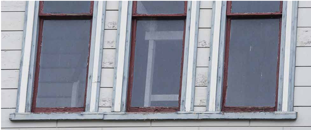
Photo 58: Windows # 46, 47, & 48 at the attic. The bottom rails of the lower sash are extremely eroded and checked, as are the lower portions of the stiles and the meeting rails. Replacement is warranted.
