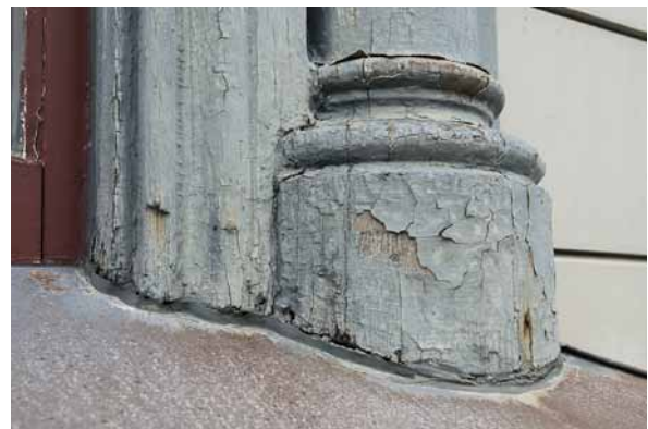
Photo 19: The turned bases to the pilasters have developed cracks and weather checking, but the sloped copper cladding on the sill prevents any leaking water.
