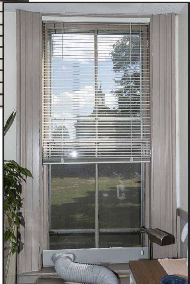
Photo 52: Interior of a typical type A window on the first floor. The tops of the window frame casings were cut and removed to install the current dropped ceiling that is present throughout the first floor. In other respects, the interior woodwork is in sound condition. Although the upper sash have functional weights and pulleys, they are not usually opened, and some may be painted shut. A number of the windows have air conditioners in the summer.
