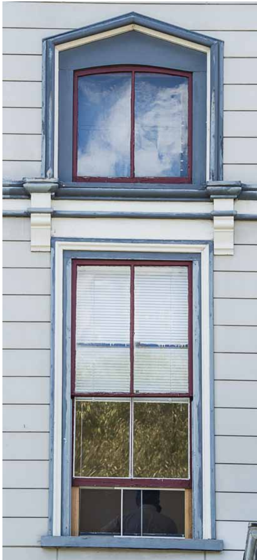
Photo 46: Windows #21 (type C) and #41 (type D, upper window) on the front facade. The sash at #41 is fixed in place. Its bottom rail has some moderate weathering. At #21, the corner joints of meeting rail of the upper sash have gaps that need to be tightened, as does the lower rail of the bottom sash. The lower rail also has a long check that needs epoxy conservation.
