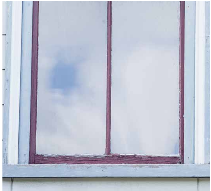
Photo 47: Windows #25 (type C) on the front facade. The bottom rail of this window has extensive checking in the bottom rail needing substantial epoxy conservation.
