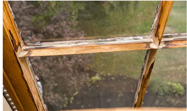
Photo 35: Detail of the knife blade profile muntins used on the replacement sash at windows #27 and 38. These windows have never been painted on their interior side.
