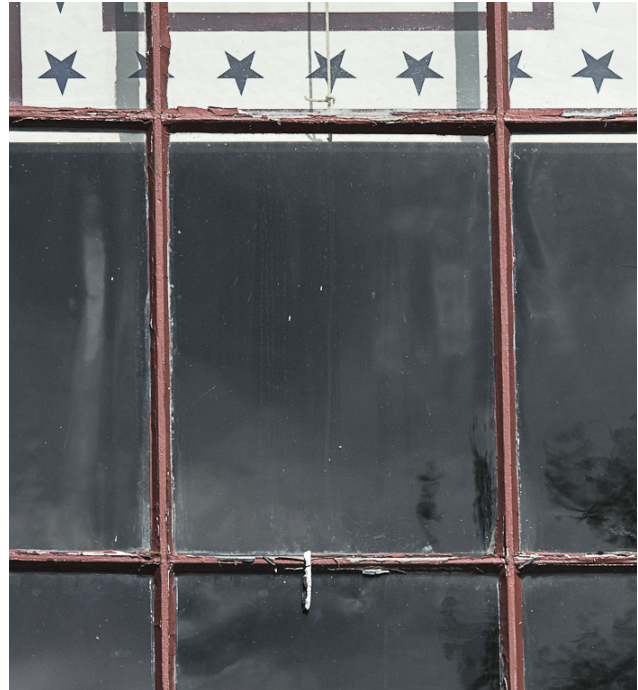
Photo 40: Detail of window #36 showing the extensive failure of its glazing compound.
