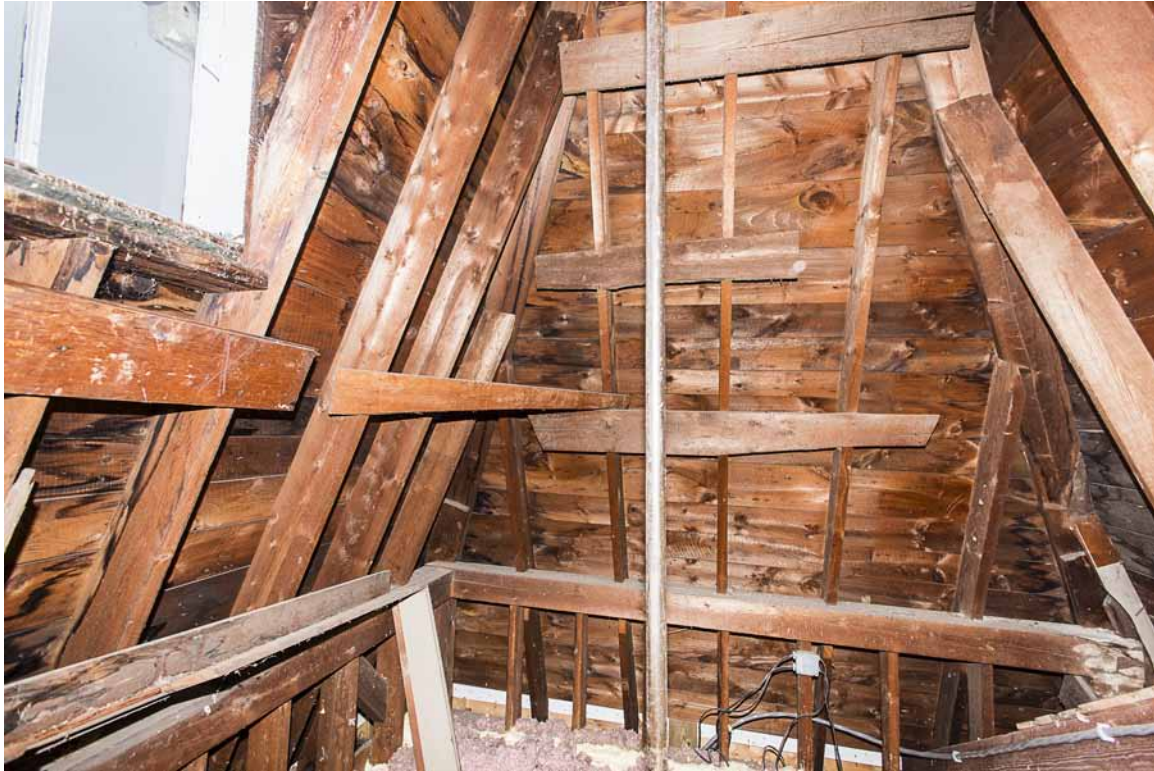
Photo90: Attic space on the south side of the center tower room looking at the sheathing on the south pitch of roof. The sheathing on the left is the front (east) pitch of the roof.
