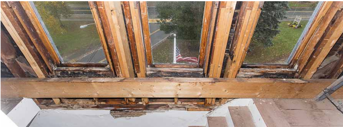
Photo 59: Interior of windows # 46, 47, & 48 at the attic. The windows leak badly during periods of prolonged wind driven rain, as evidenced by the stains below them. They have never been painted and also lack proper interior stops. The large beam is from past structural reinforcements to the tower.
