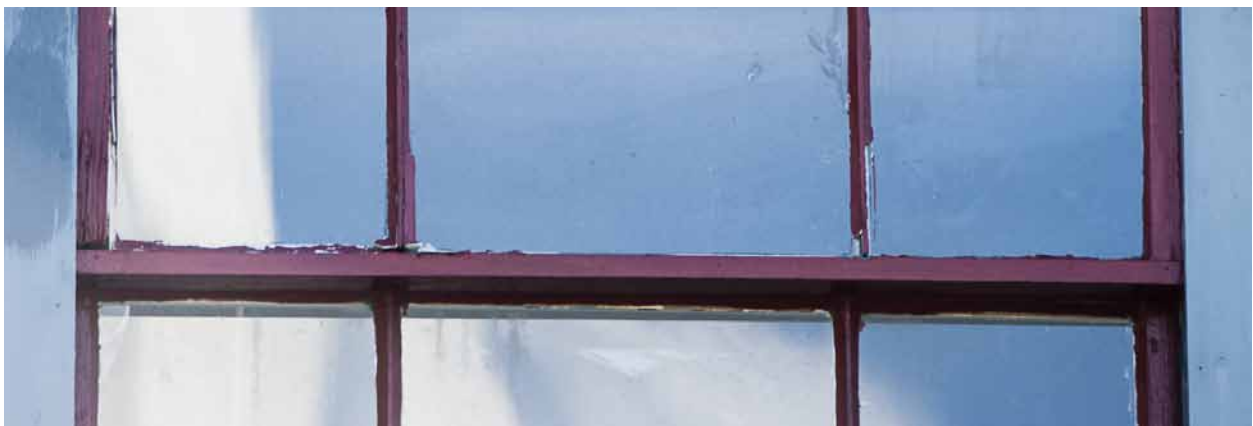
Photo 36: Detail of the meeting rail of window #27. The meeting rail of the upper sash has dropped about 1/4" on its left side, and the left stile above it has extensive splits. The meeting rail dropped off completely since this photo was taken.
