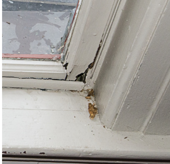
Photo 15: Detail of window 23 showing its badly rotted lower corner. The rot seems to be from a combination of water running down its stile and leaks from the turned base shown in Photo 13.
