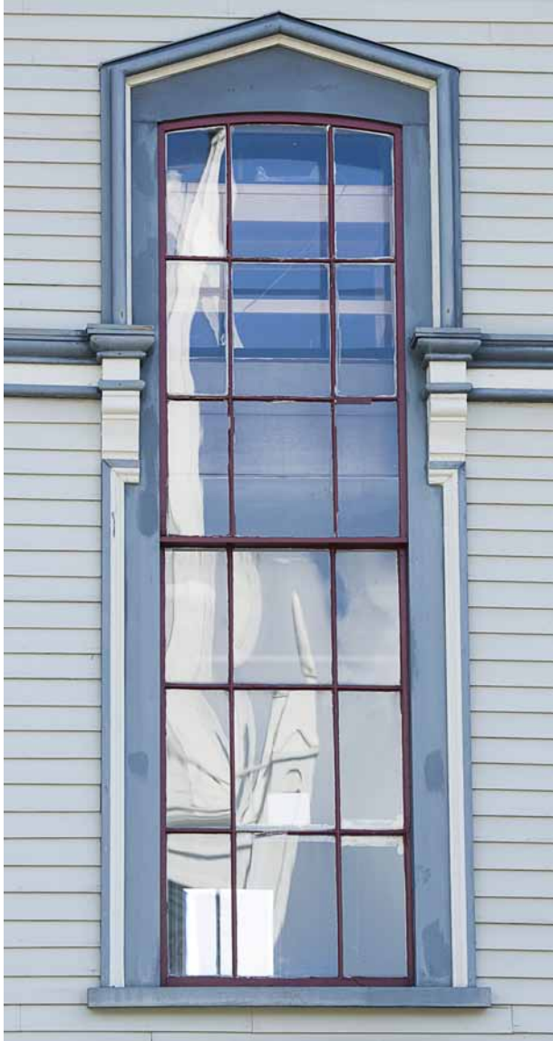
Photo 34: Window #27 on the north facade. The upper sash is a 30± year old replacement, while the lower sash appears to be original. Both have serious condition problems. The muntins of the upper sash are very thin with a knife blade profile that does not match the original sash and result in an excessively weak sash.
