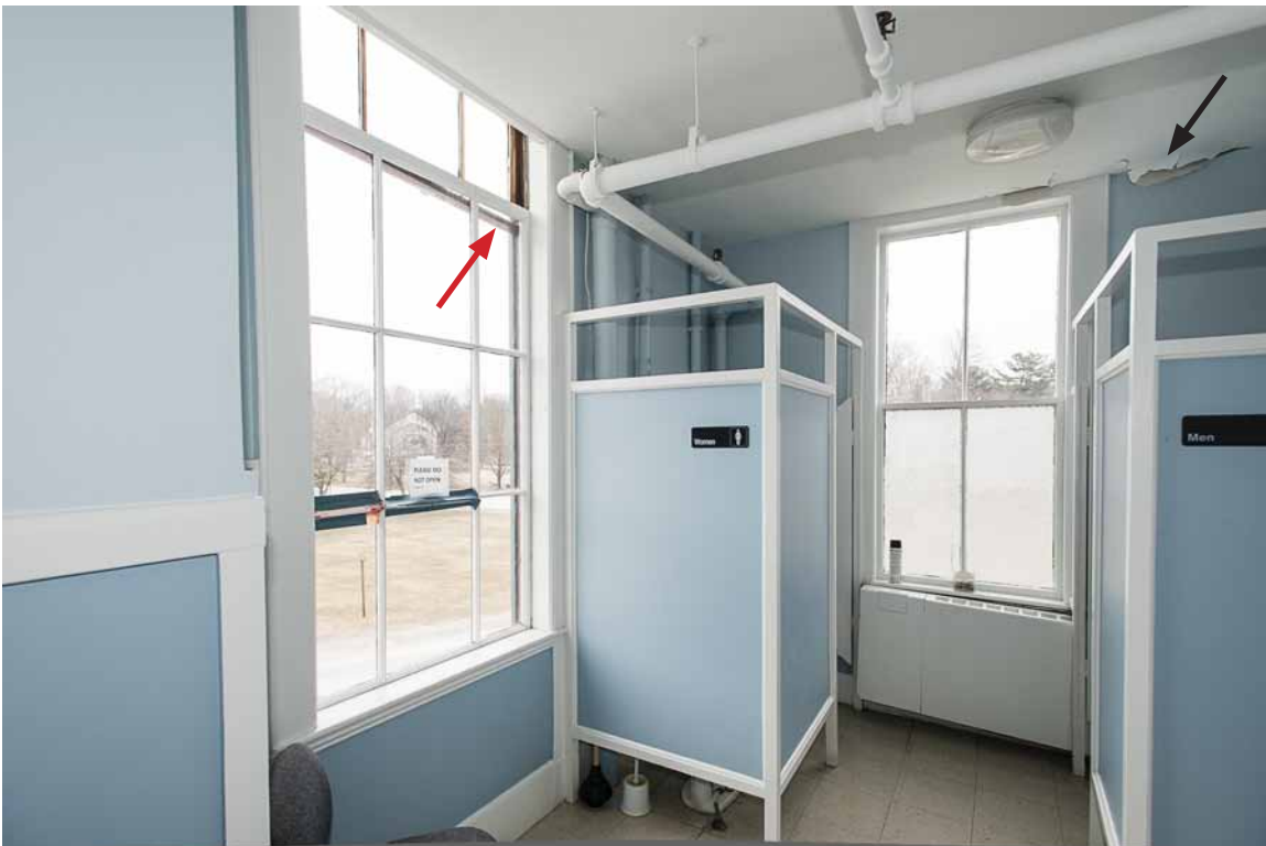
Photo 76: Northeast room on the second floor now used as a bathroom. The red arrow points to the upper sash meeting rail which has dropped down substantially from its original position (Window #27). The black arrow points to peeling paint from a past leak that is not believed to be current.
