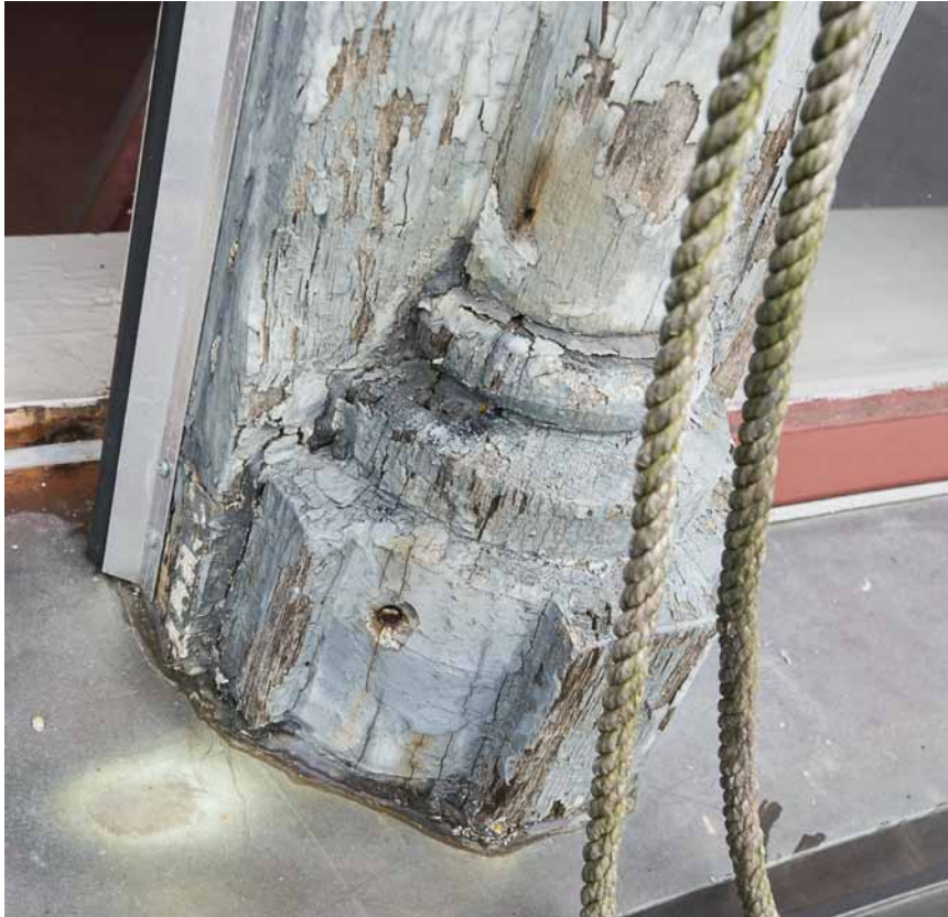
Photo 12: Turned base to the pilaster between windows 23 & 24 has splits and weather checks that allow water penetration under and behind it. Caulking at its bottom traps any water that gets behind it.
