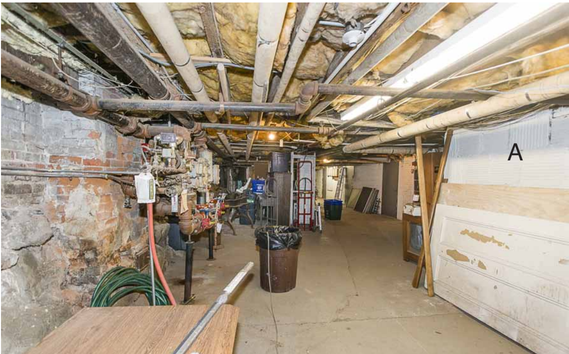
Photo 99: Basement looking east towards the front of the building. The north side foundation wall is on the left. The ceiling has been insulated with fiberglass batts. "A" marks a terra cotta block wall that encloses storage rooms and some utilities. Although concerns have been expressed that mold is present in the basement from past leaks and basement dampness, no evidence of current mold was observed. The exposed fiberglass presents some risk of airborne fiberglass particles, and also could conceal unknown deterioration of the framing. The pipes are insulated with foam.
