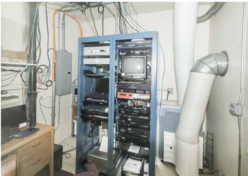
Photo 85: Room in the northeast corner of the balcony level that is now used by the local cable station. The room is heavily insulated with new walls inboard of the original walls and kept at a constant temperature with its own HVAC equipment.
