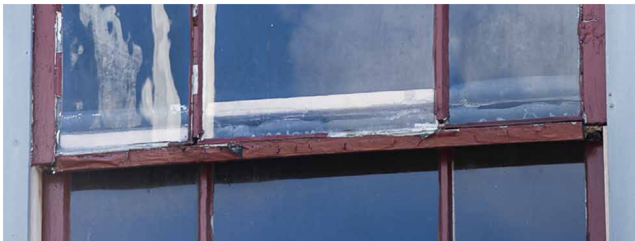
Photo 38: Detail showing the dropped upper sash meeting rail of window #32.
