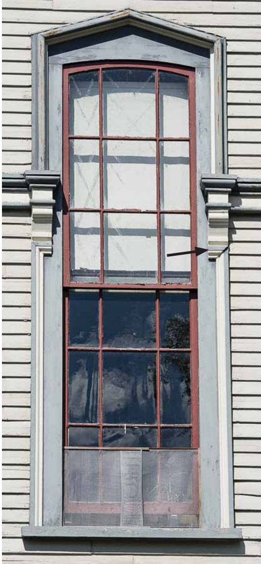
Photo 39: Window #36 on the south facade. Its condition is typical of most of the type B windows on the second floor. Its glazing compound is badly deteriorated, but it retains most of its original glass. The corner joints of the upper sash meeting rail remain sound. The lower rail of the lower sash has some moderate weather checking that warrants conservation with epoxy consolidants. The arrow points to a loose molding that needs to be renailed.
