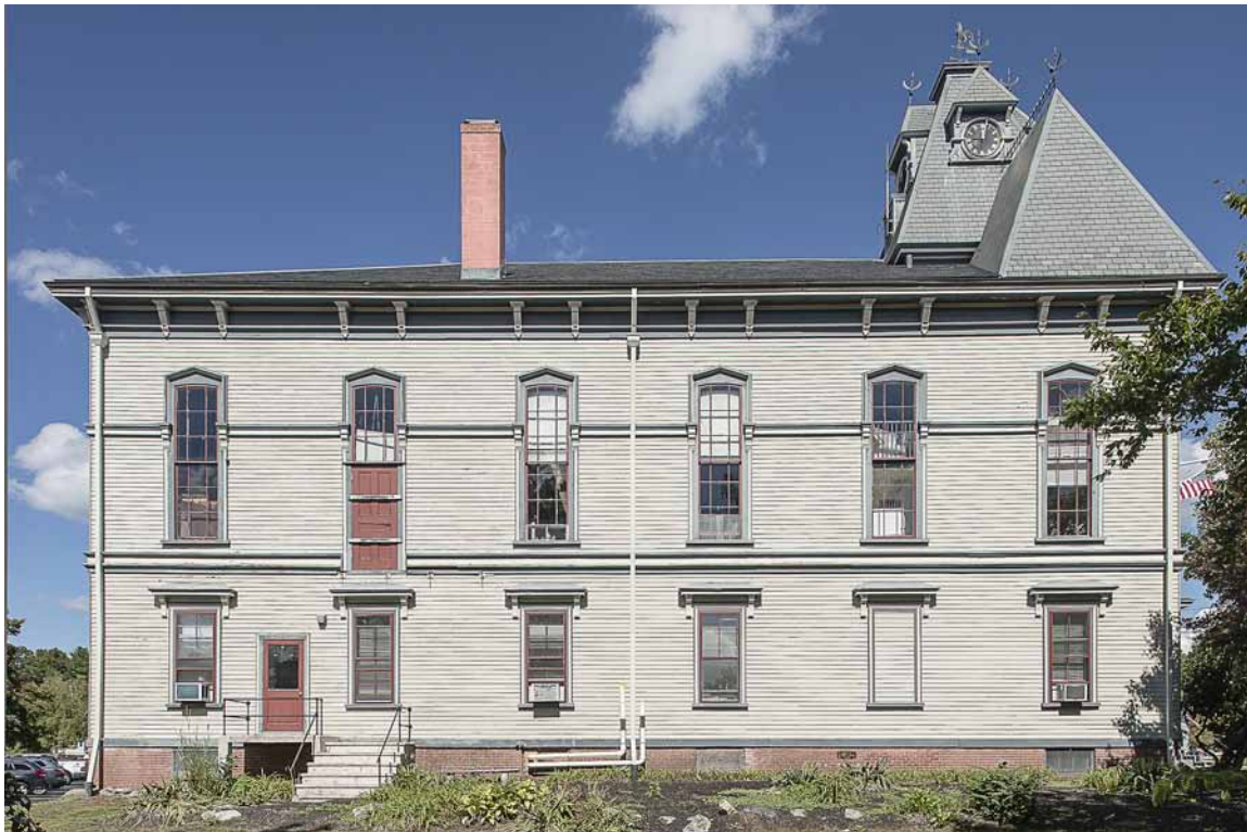
Photo 6: South facade. Clapboards are original; no work was done to this facade in 2003. The foundation has some areas of open mortar joints that need to be cut out and repointed.
