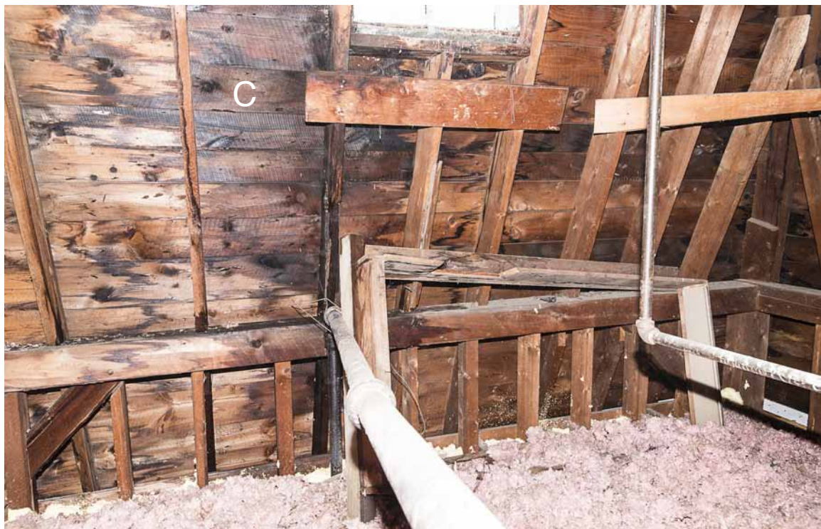
Photo 91: Attic space on the south side of the center tower room looking at the sheathing on the front (east) pitch of the roof with window #49 in the upper center. This photo was taken the same day as #87. The wet area at "C" is from the flashings on the east side of the dormer roof of window #49. Like the leaks in photo 89, they only occur a few times a year and do not appear to be affecting the floors below.
