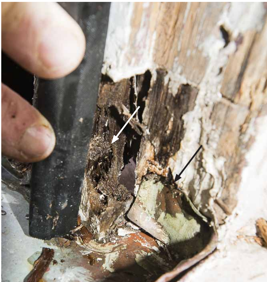
Photo 16: Detail of the bottom of the right side jamb of window 23 showing wet and rotted wood (white arrow) and poor flashing detail (black arrow) that allows water to flow behind the flashing and into the structure below.
