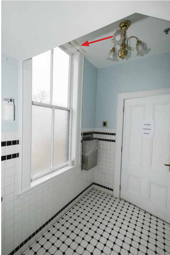
Photo 71: First floor bathroom that has been renovated to provide an handicapped accessible bathroom. The water stains above the window (arrow) are from leaks through the badly deteriorated window #32 directly above.
