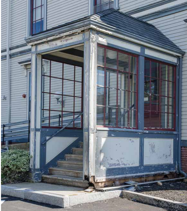
Photo 20: The westerly entry “doghouse” porch that was installed in 1995 (??) shows extensive rot of both trim and framing causing it to be removed last December due to concerns it might collapse under heavy snow. The easterly doghouse is only slightly better and will likely be removed this spring.
