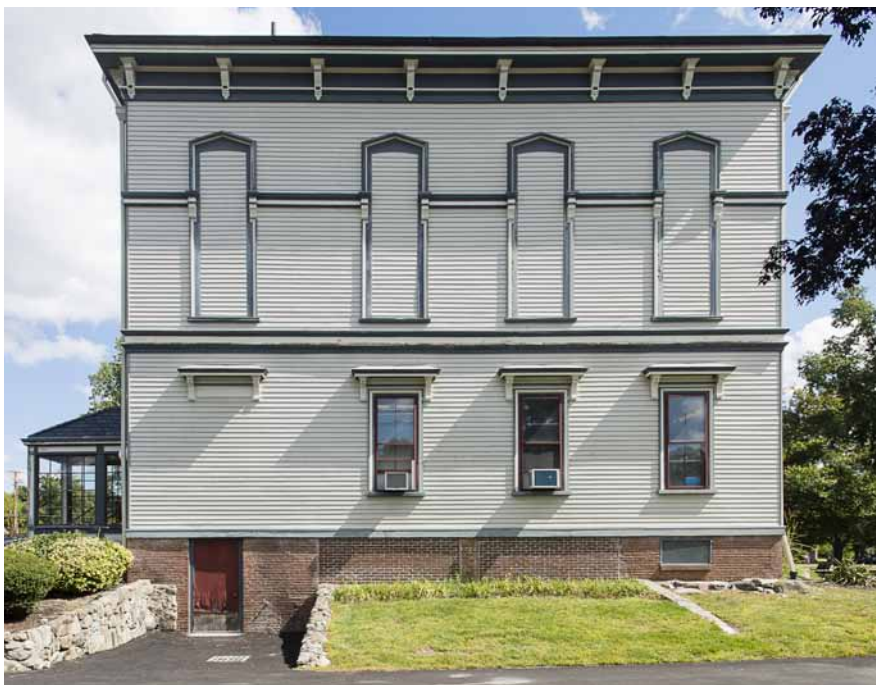
Photo 4: Rear (west) facade. All the clapboards were replaced in 2003. The bricks at the foundation of this facade have numerous open or otherwise defective joints and should be 100% cut and repointed with a high lime mortar compatible with the relatively soft brick used in the foundation. Refer to photo 15 for a detailed view.
