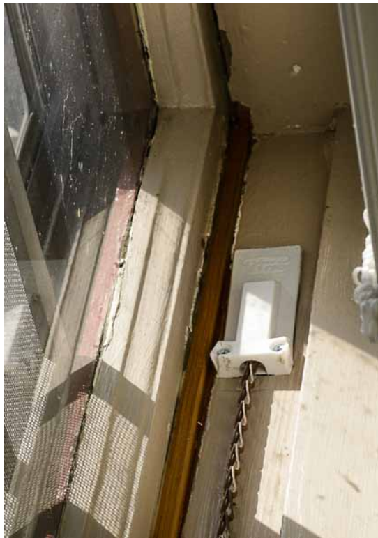
Photo 55: A number of the pulleys on the first floor have been replaced with modern pulleys and new chains. While not original, these are serviceable. The parting bead of this window has also been replaced.
