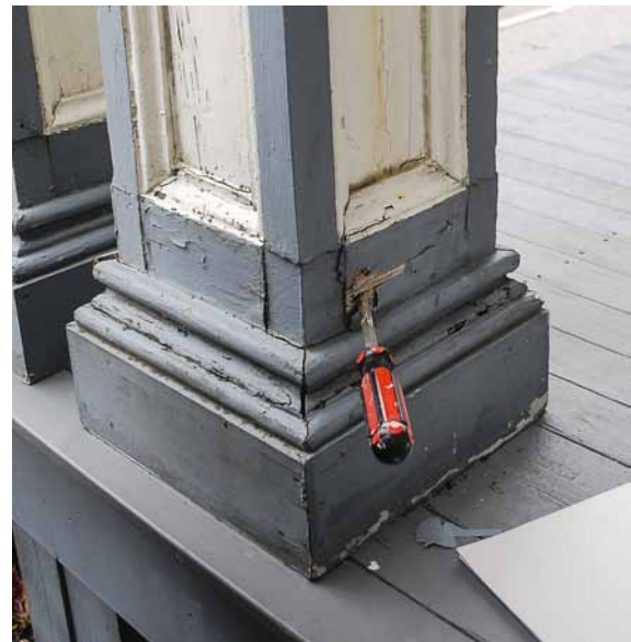
Photo 9: Some of the trim on the lower portions of the columns are rotting.
