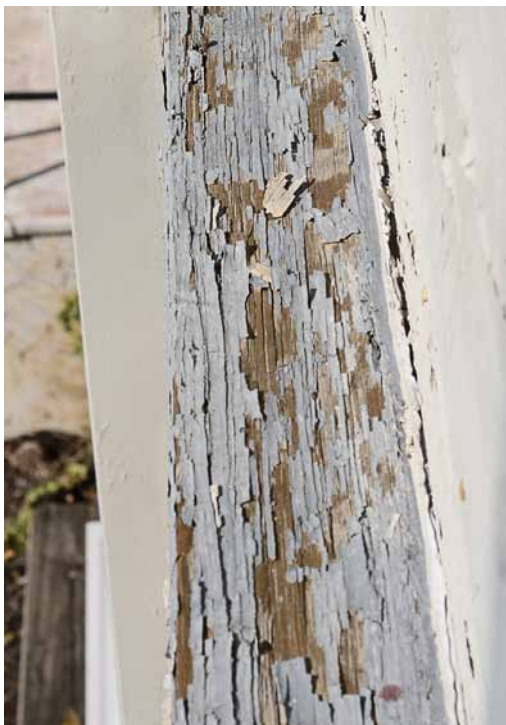
Photo 25: Top surface of upper belt course on south side has extensive paint failure and moderate weather checking. A few areas have deeper weather checking. Despite the checking, the wood remains sound and hard, including within the checks.
