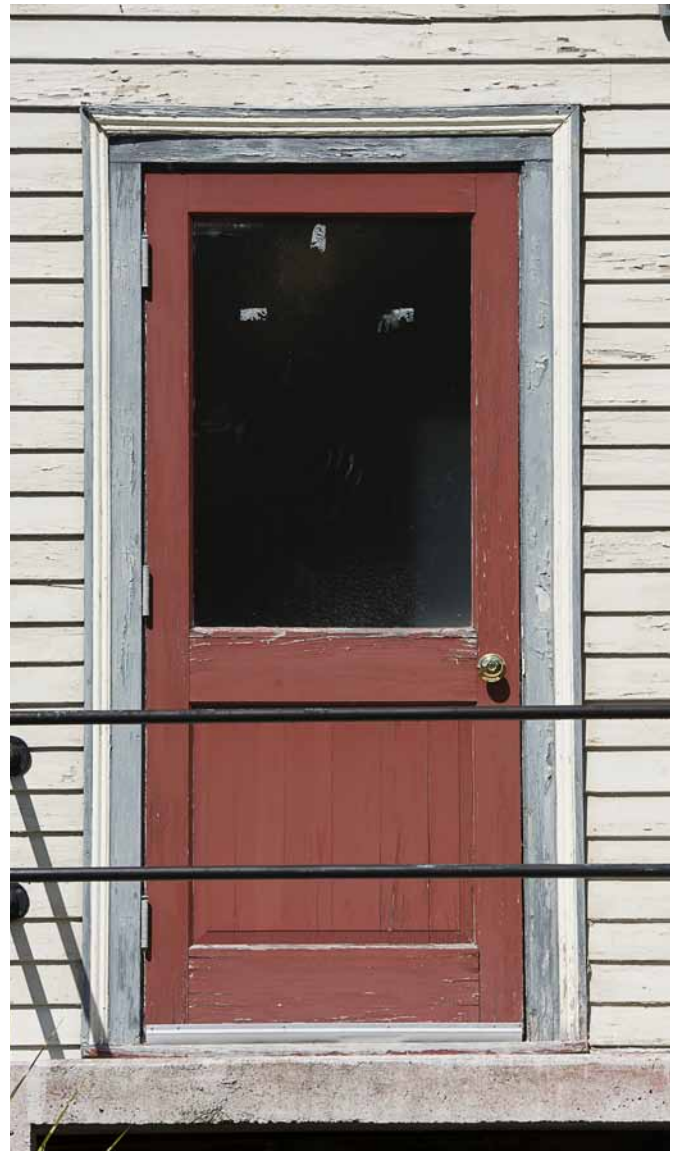
Photo 27: Egress door from a south side office on the first floor. The lower panel of the door is developing splits at its laminations.
