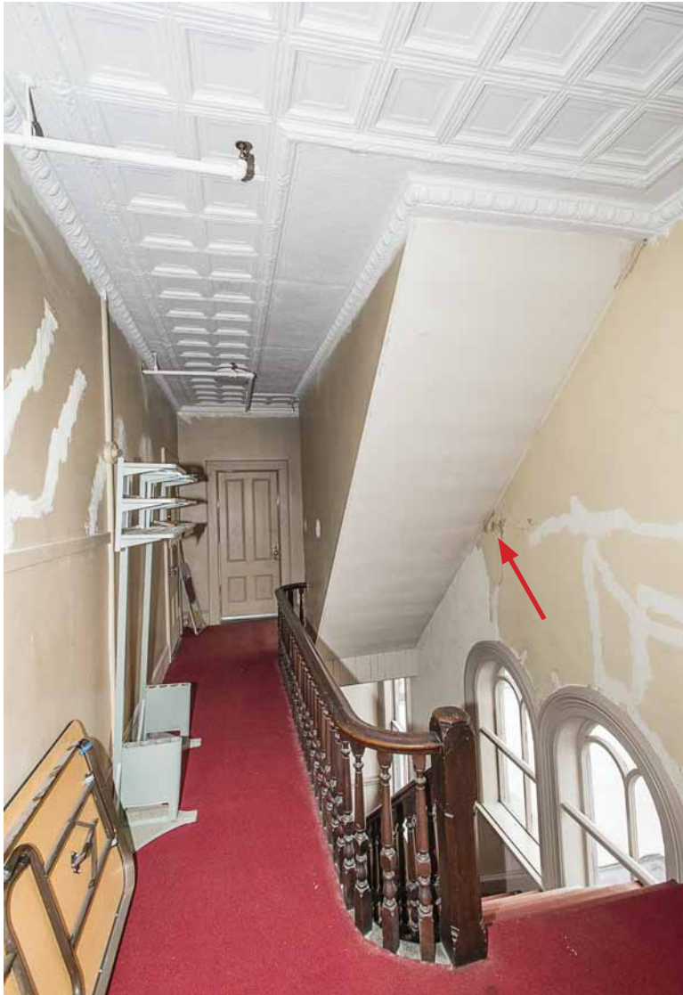
Photo 84: Hallway behind the meeting hall balcony with stair down to the second floor. The stair at the rear of the photo leads up to the attic and the clock tower. The arrow points to old water damage that is not from current leaking. The white patches cover plaster cracks from past structural movement of the tower that was stabilized with reinforcements some years ago.
