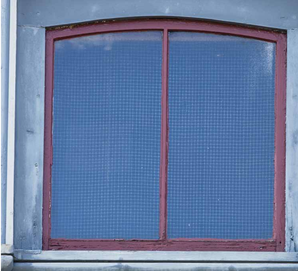
Photo 49: Window #44 (type D). Its bottom rail has fairly severe weather checking and 1/8" gaps at the corner joints, but the sash is other sound.
