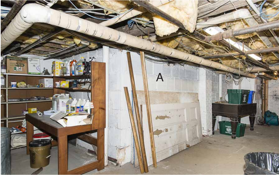
Photo 100: Basement looking southwest with the rear wall at the extreme left of the photo. “A” marks the same terra cotta block partition marked in photo 99 above.
