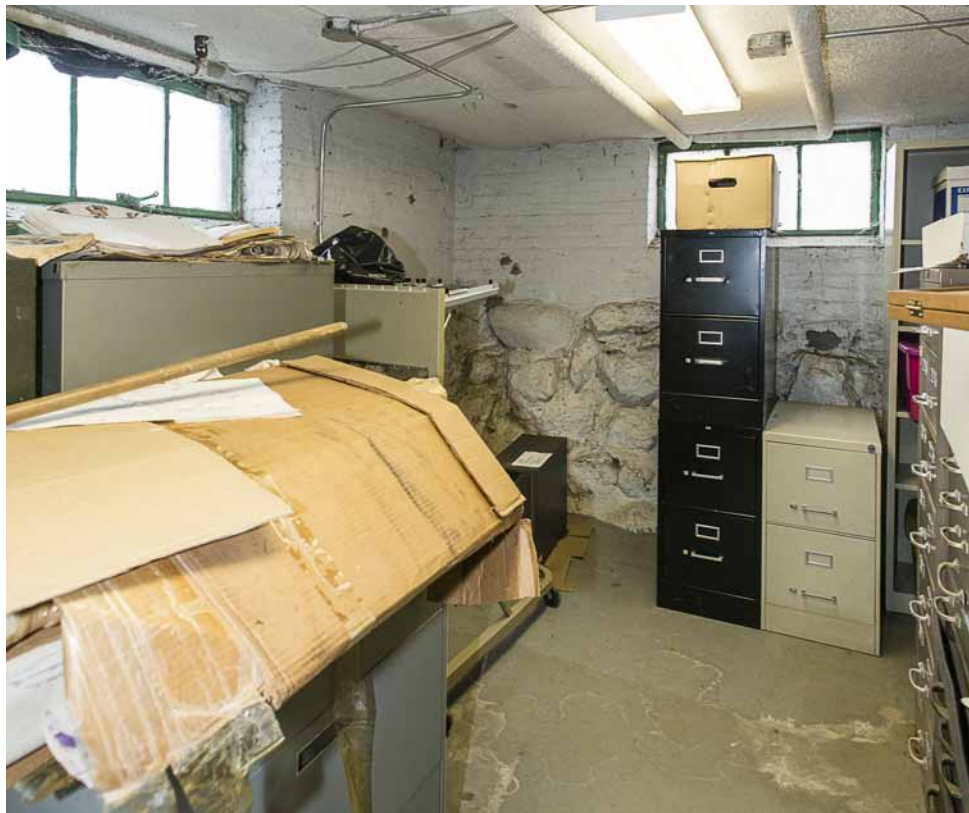
Photo 101: Southwest corner of basement showing typical document storage use. The brick portion of the foundation wall is above grade. The south wall is on the left. Some water stains are visible on the floor from past dampness.
