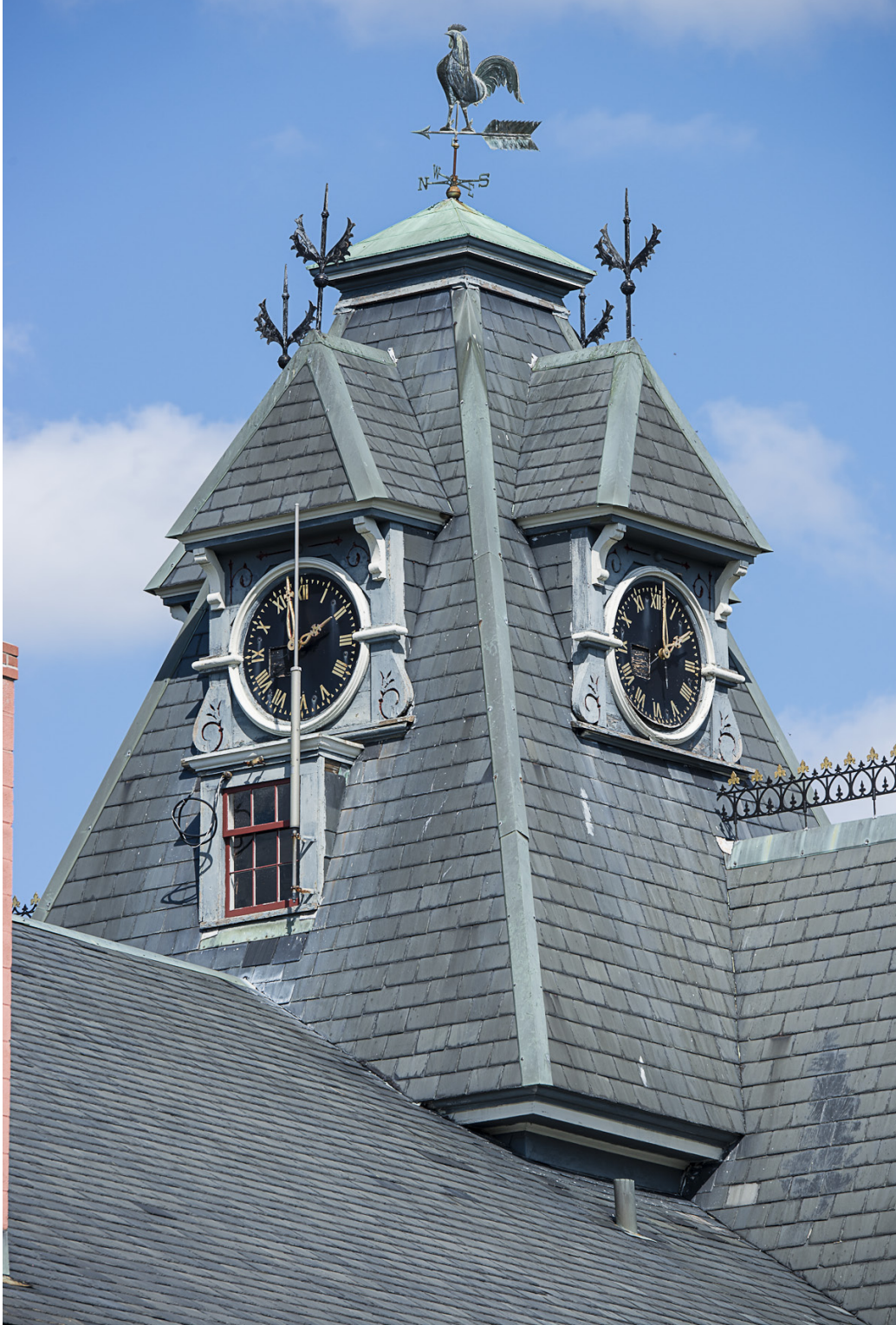
Photo 33: Overview of rear (west) and south sides of the clock tower. The woodwork appears to remain sound other than peeling paint. The slate also appears sound. Although no leaks are known to occur from the closed valley flashings on this side, their condition is probably have similar to the valleys on the northeast side.
