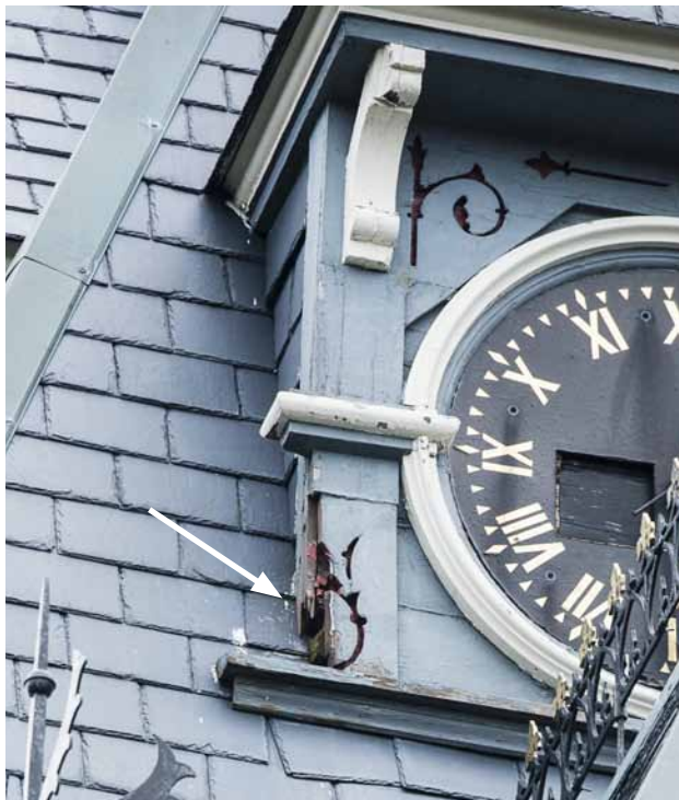
Photo 30: Rotted area of wood decoration at the clock tower marked with the white arrow in photo 28. Trim at the other clock faces appears to remain sound.
