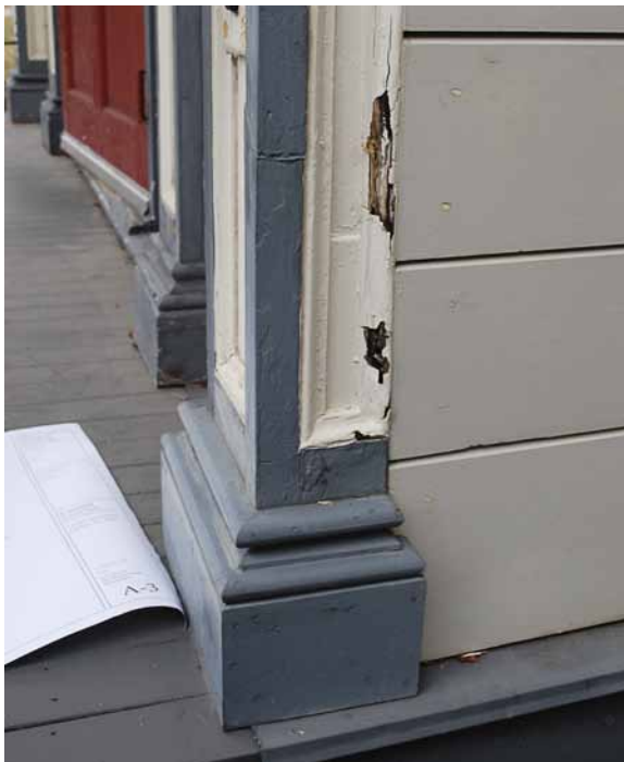
Photo 8: Many of the trim elements are rotting.
