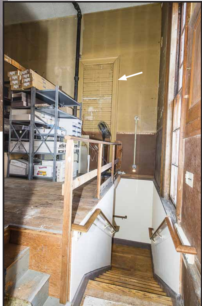
Photo 80: Stair at the north end of the stage area has been recently renovated to provide a second egress for the offices in the meeting hall. One of the blind windows in the rear (west) wall is visible in the center of the photo (arrow). It is not known these windows ever contained glazed sash. Window #32 is on the extreme right.
