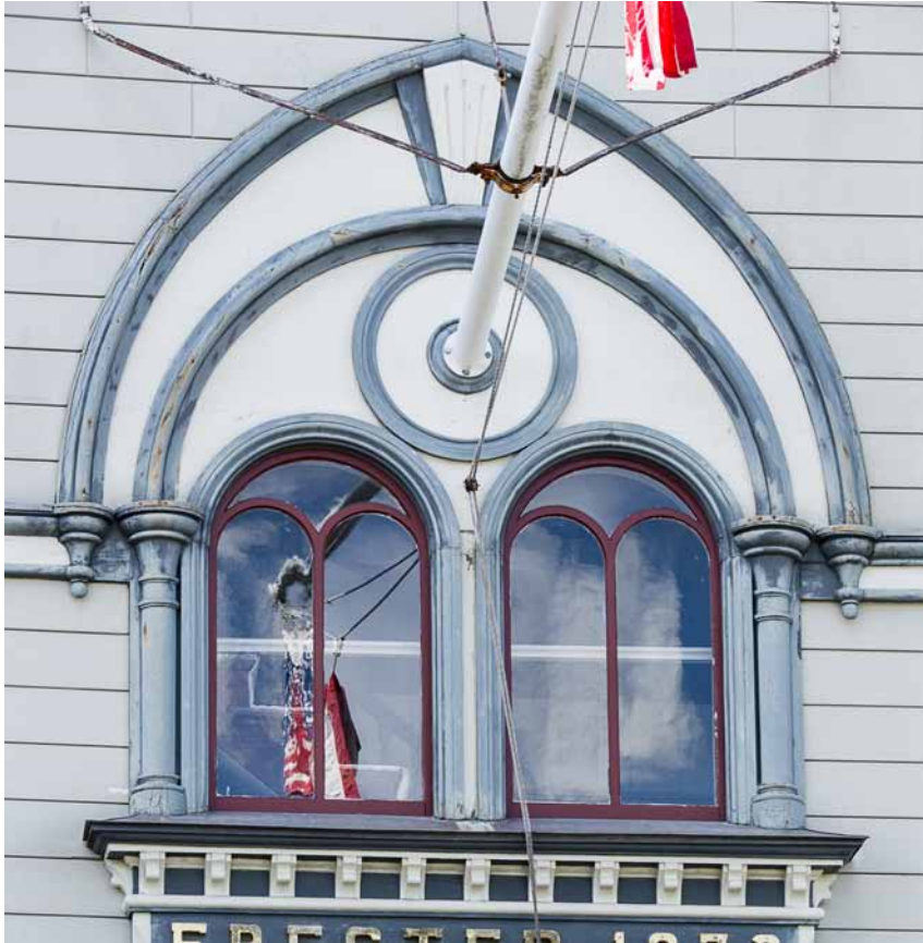
Photo 17: Windows 42 and 43 and related trim. The window sash remain reasonably sound with minor glazing defects.
