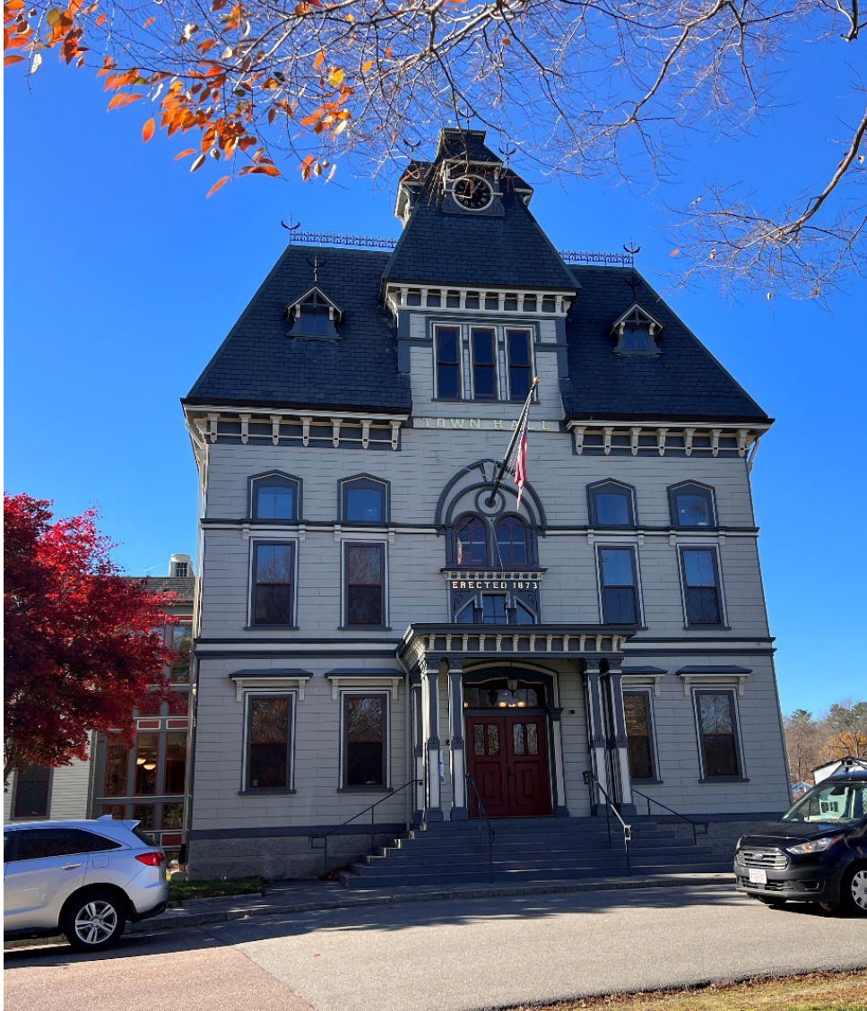
Town of Topsfield Town Hall, Source: Elana Zabar, 2022.
