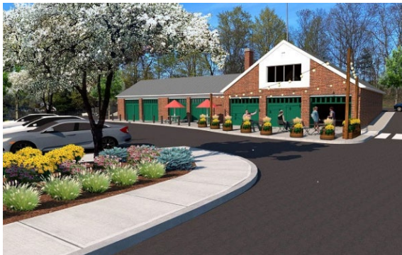
Topsfield Highway Garage, Source: Topsfield Town Website.
