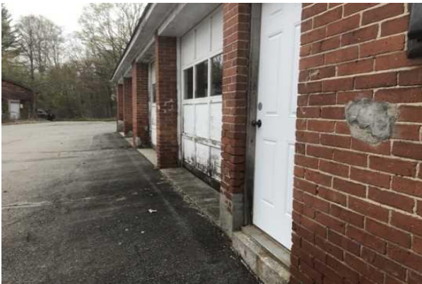
#11 DAMAGED BRICK VENEER
