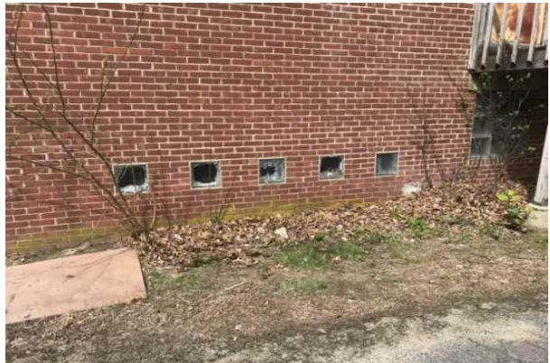
#10 BROKEN GLASS BLOCK OPENINGS
