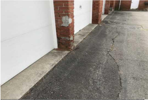
#13 DAMAGED PILASTERS AT GARAGE DOOR OPENINGS
