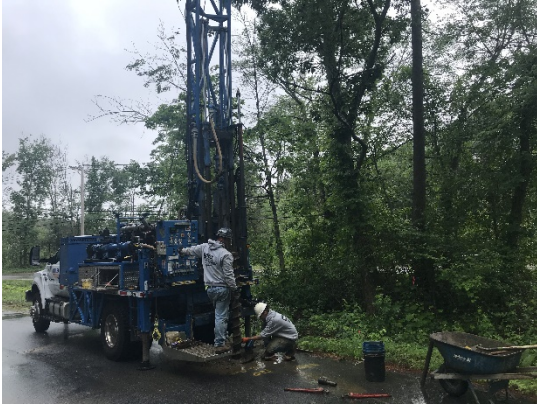
Drill Rig Setup
