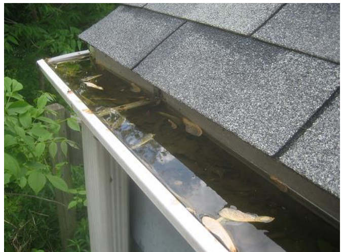
Figure 8. Clogged rain gutter filled with water
